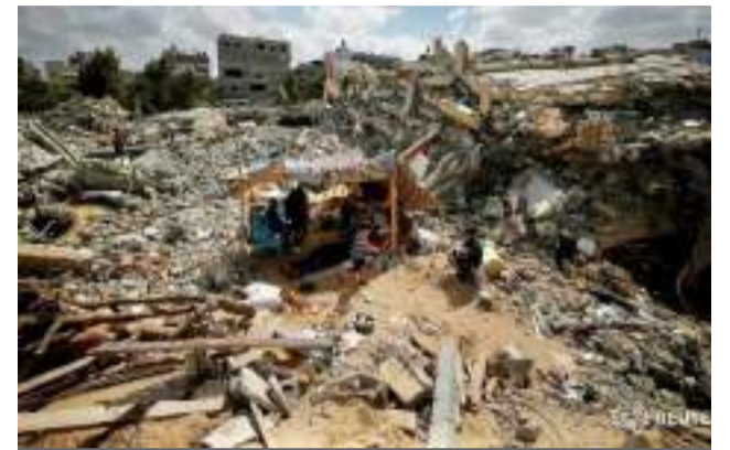
The bombing has damaged several buildings and structures in Gaza strip
